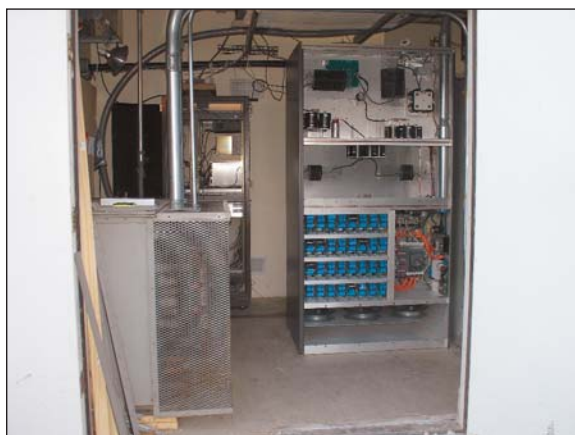
After installation – a comfortably tight fit.
