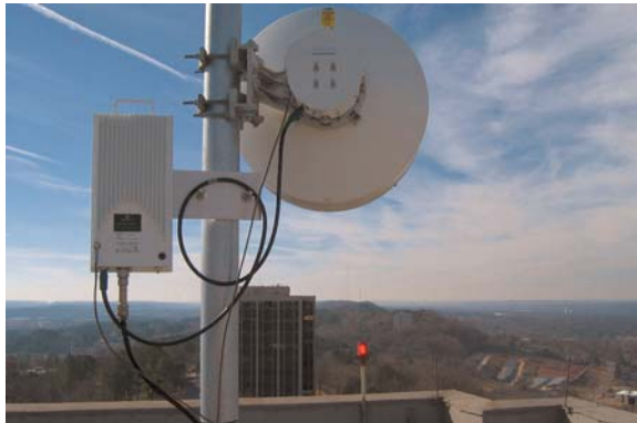
A Dragonwave Airpair 18 GHz link got the data stream to the transmitter.
